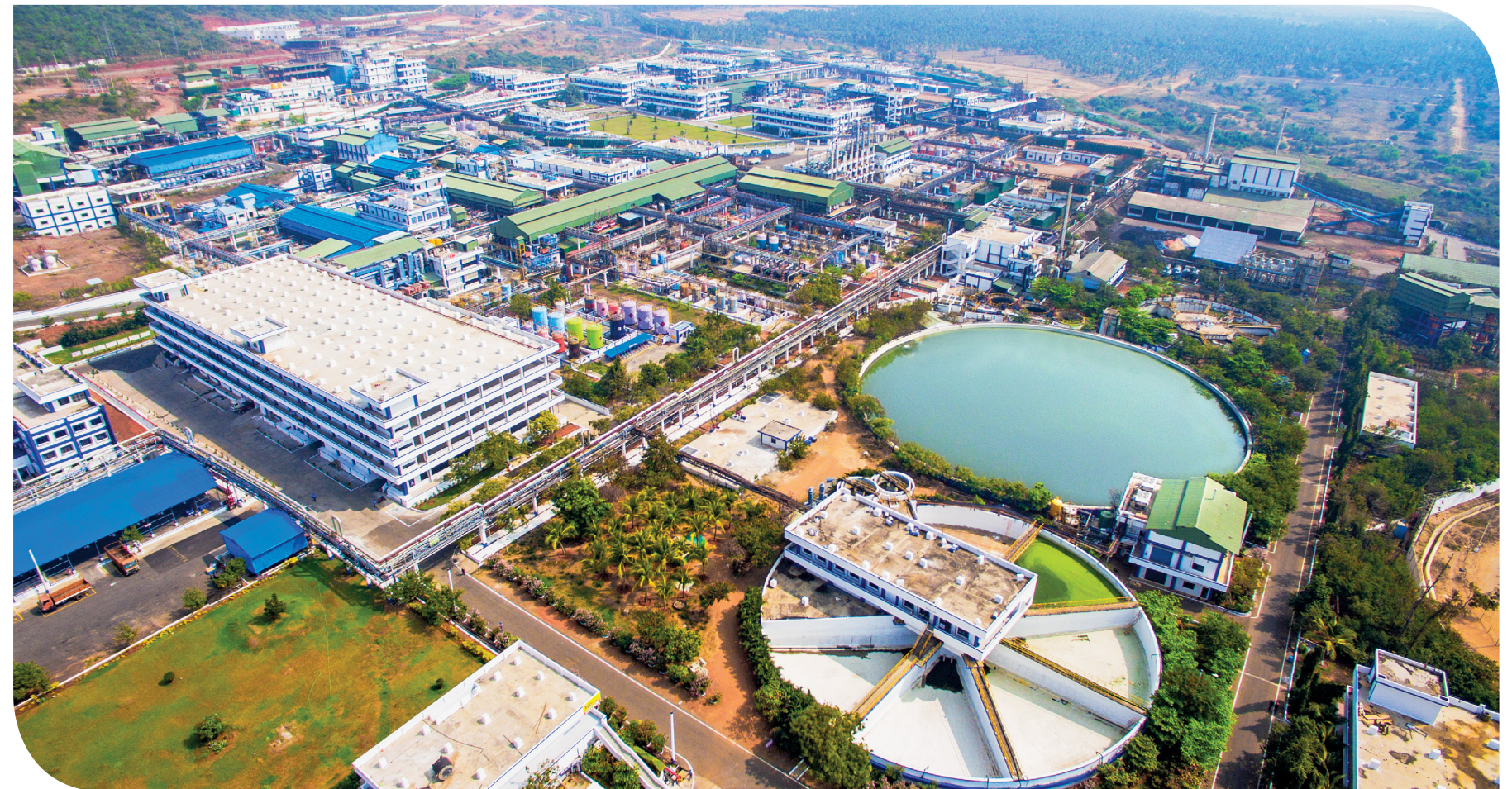
Aerial view of the manufacturing facility in visakhapatnam
