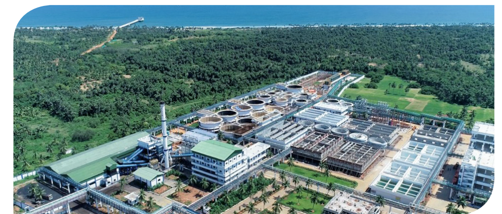
State-of-the-art, Off-ground Effluent Treatment Plant, facilitating a sustainable operating environment - Unit 2, Visakhapatnam
