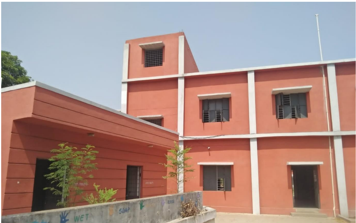
Pic 5 - Toilets & new building
