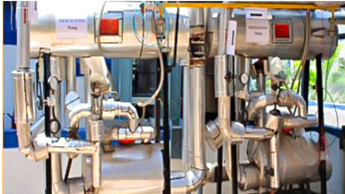
Installed packaged pressure powered pump unit (PPPPU)
