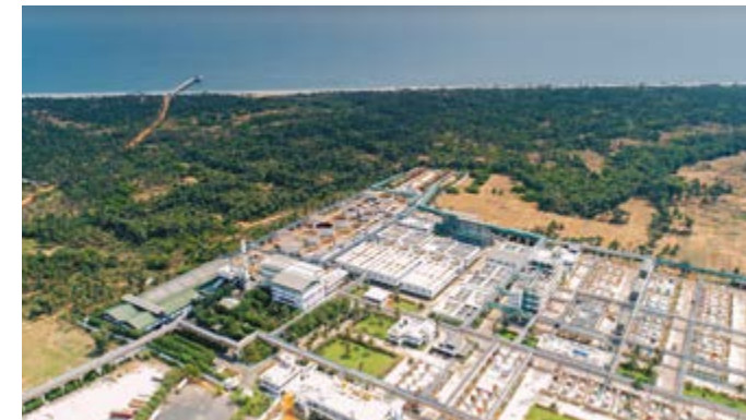
Off-the-ground effluent treatment plant
