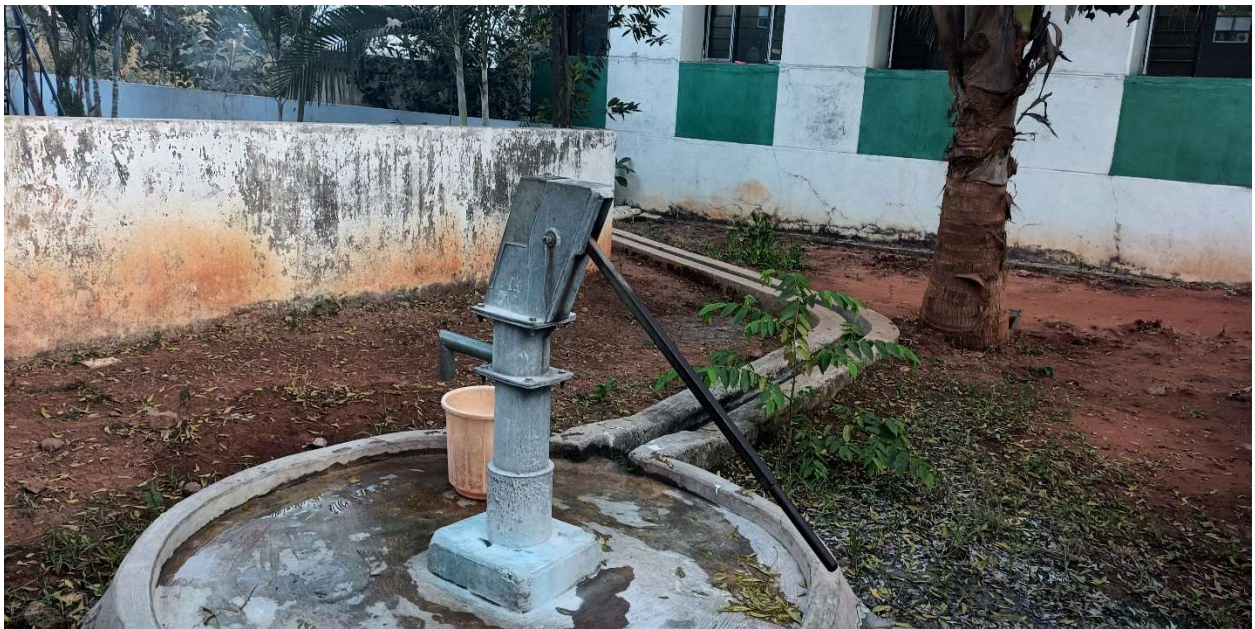
Pic 8 – Platform around the Handpump & Water Draining Channel
