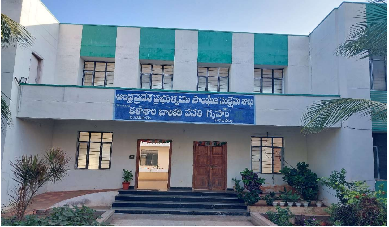
Pic 1 – Social Welfare Hostel Building at Paradesipalem
