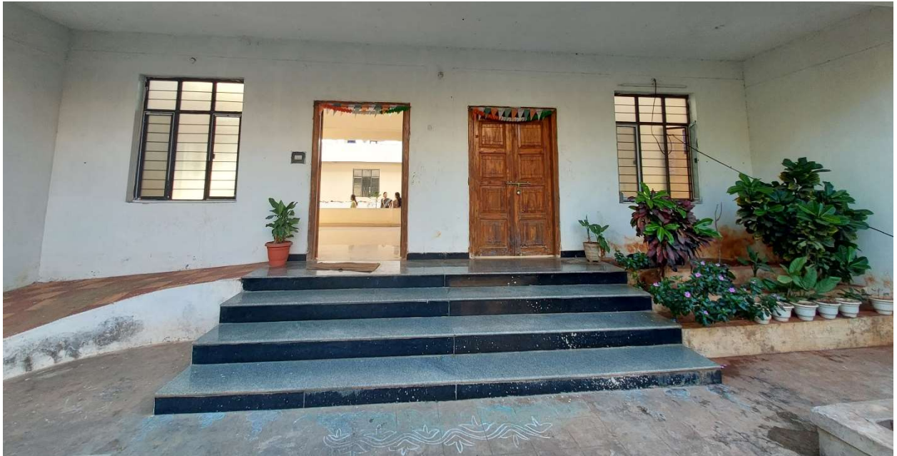
Pic 2 – Ramp and Steps leading into the Hostel
