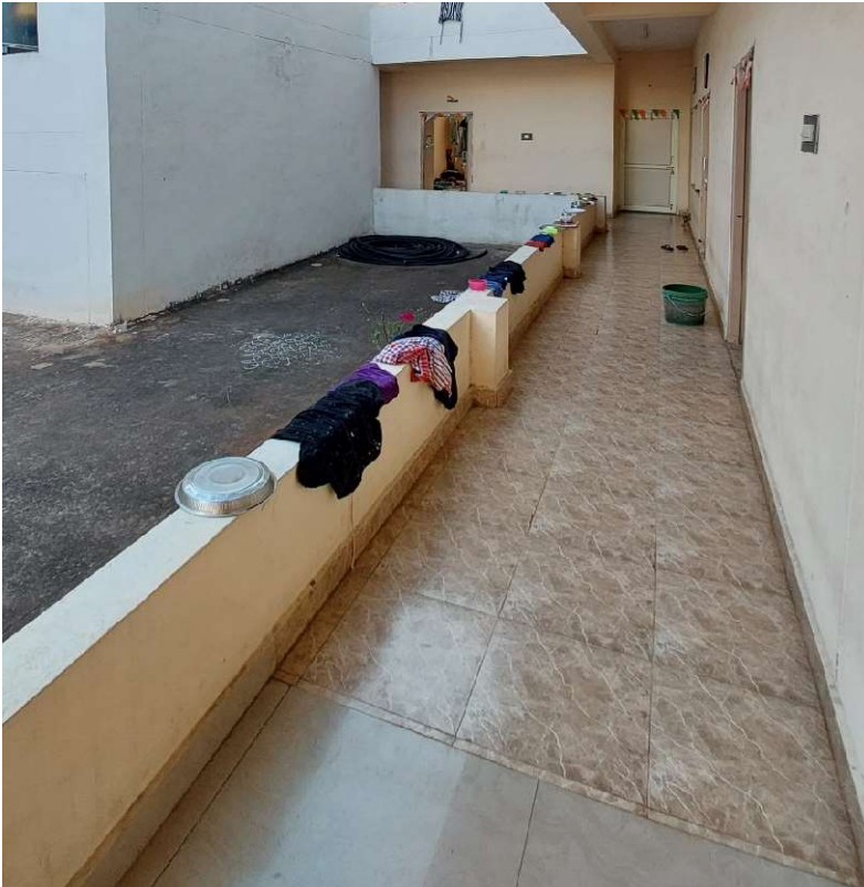
Pic 6 – Tiled Flooring in the Corridor in front of the rooms
