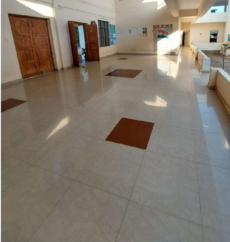
Pic 5 – New Flooring with Vitrified Tiles inside the Hostel
