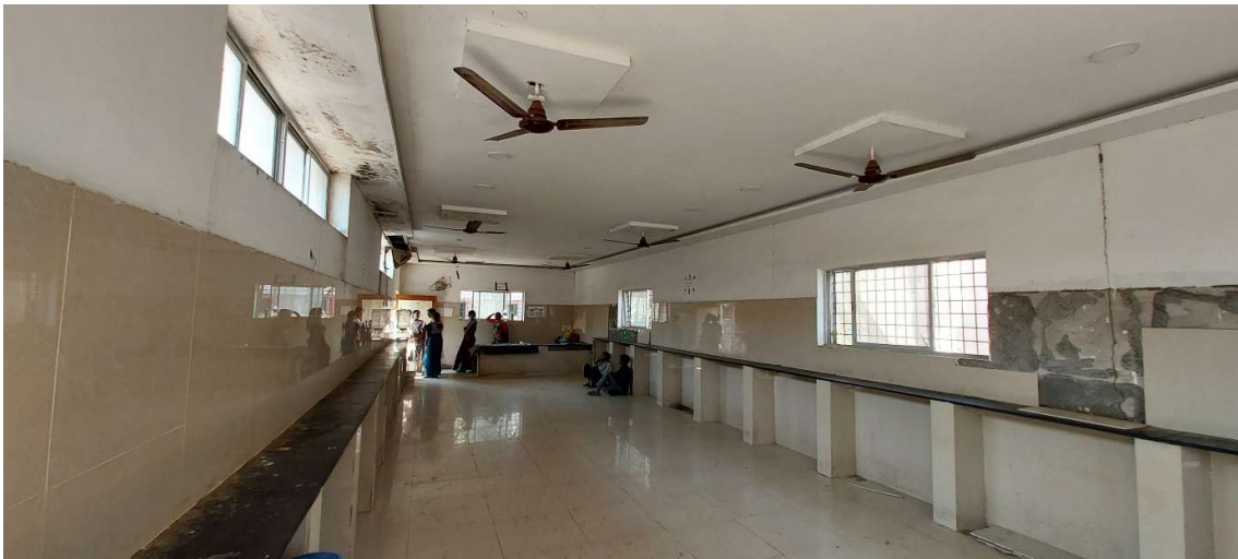
Pic 7 – Renovation work in Annapurna Canteen
