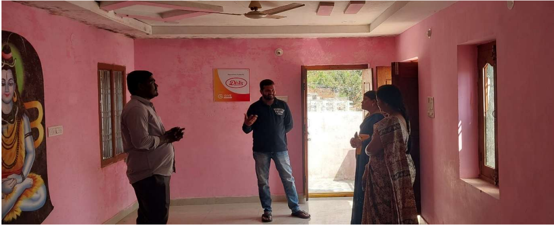
Pic 6 – Repair work taken up at the Urban Shelter
