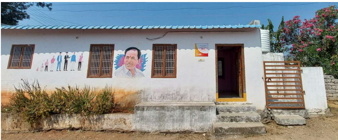
Pic 5 – Construction of Gate and Toilet in the community hall
