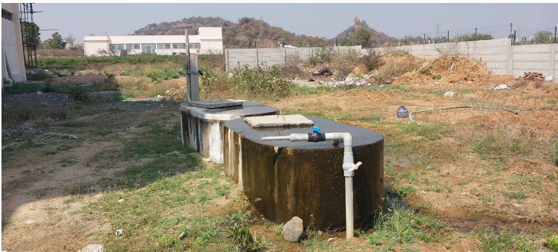
Pic 8 – Water tanks each 5000 litres capacity at KGBV Rajanna Siricilla
