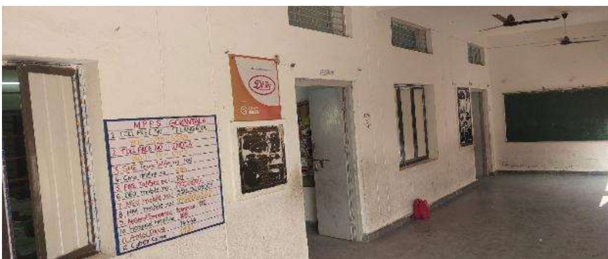
Pic 5 – Wide verandha in front of the classroom in Gorantala MPPS
