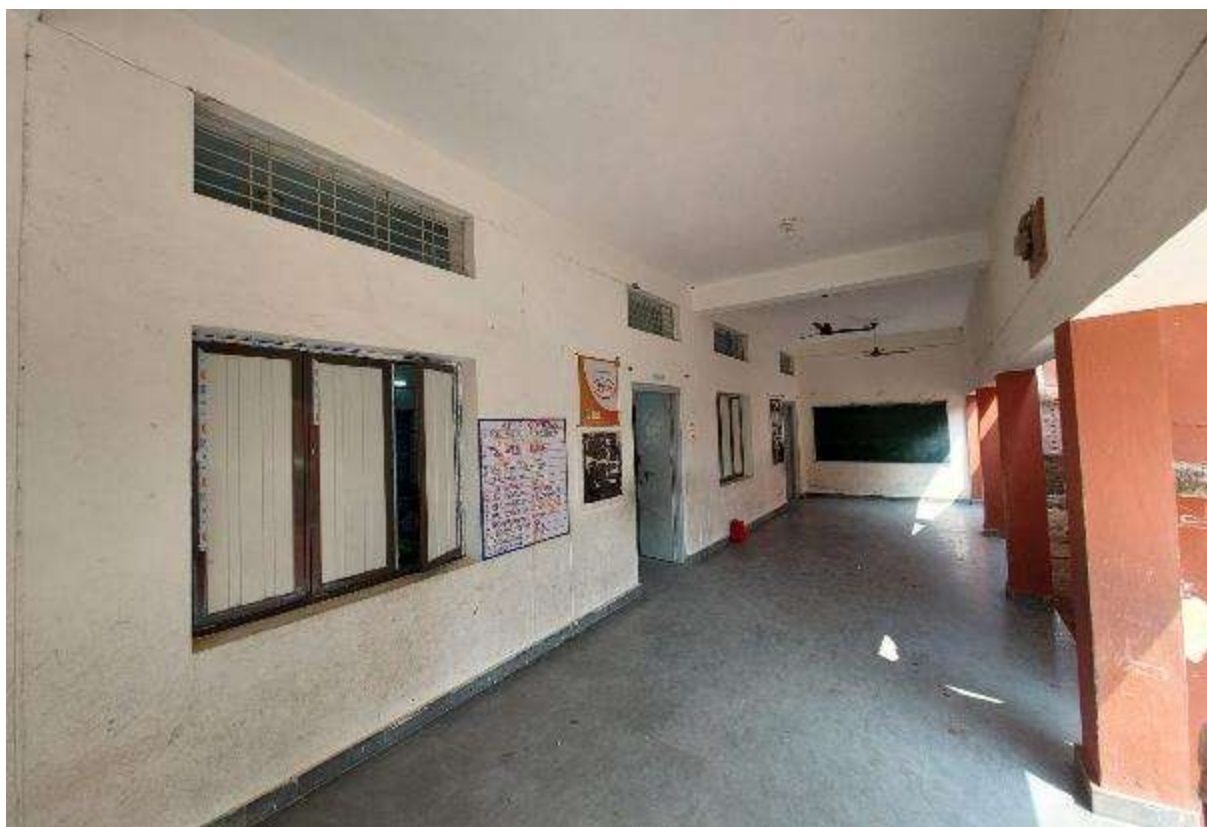
Pic 2 – Construction of a new school building block at Gorantala
