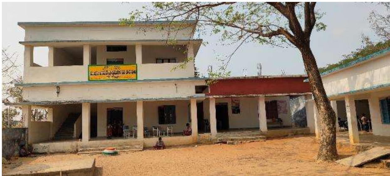
Pic 1 – Construction of an additional school building block at Narmola
