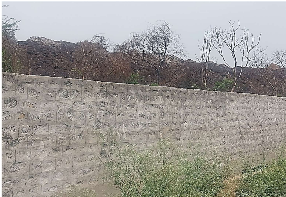
Pic 7 – Trees affected by chemical contamination from nearby industrial effluents
