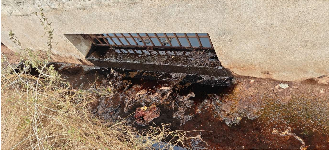
Pic 4 – The iron grill mesh at the base of the compound wall to prevent large waste materials from entering the drain
