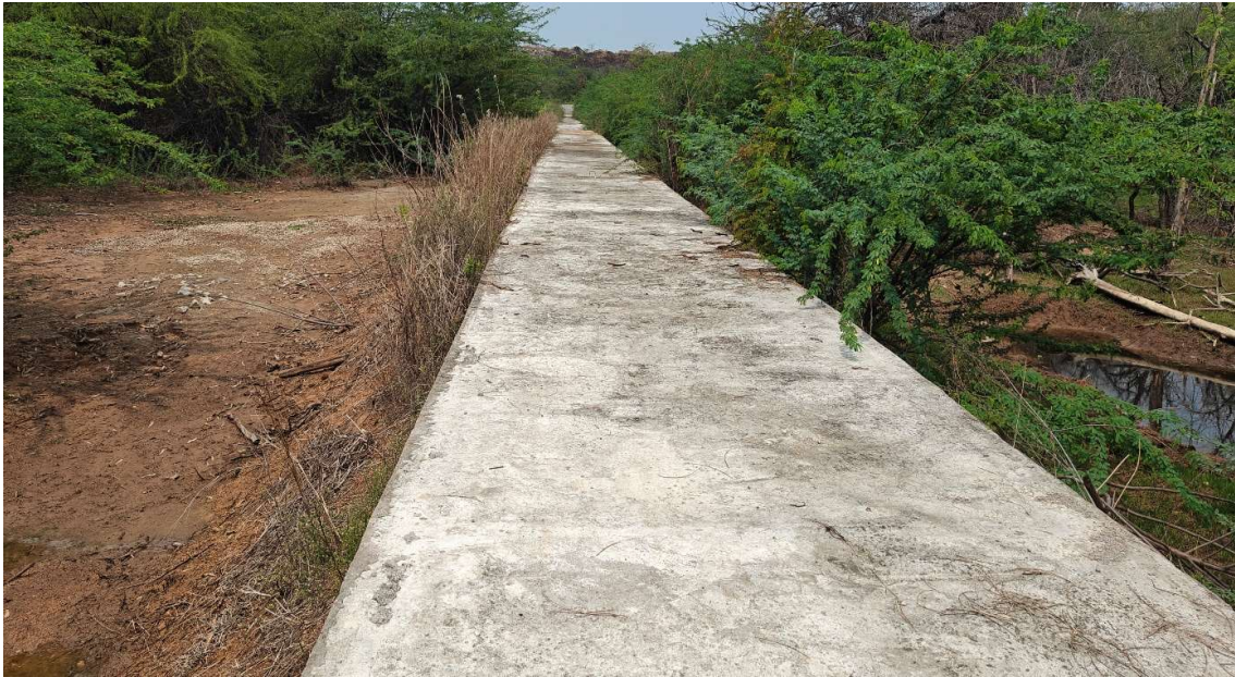
Pic 2 – The newly constructed 22- meter-long box drain
