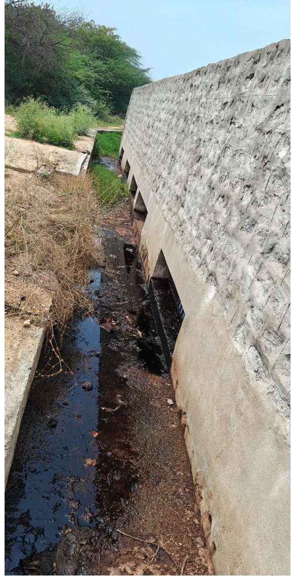
Pic 8 & 9 – Drainage canal constructed along the compound wall inside to channelise rainwater runoff into the box drain
