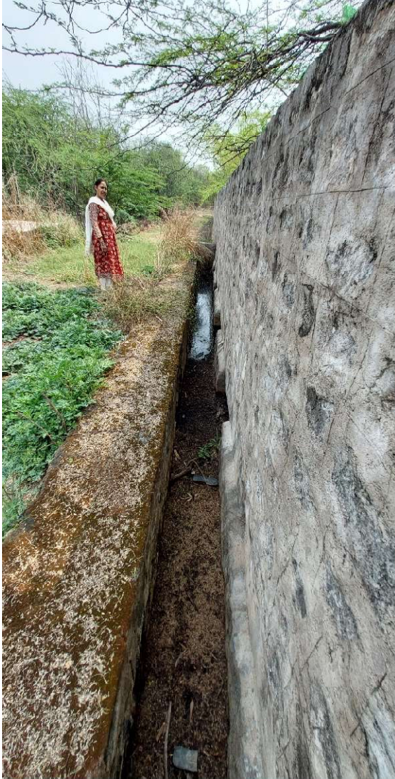
Pic 8 & 9 – Drainage canal constructed along the compound wall inside to channelise rainwater runoff into the box drain
