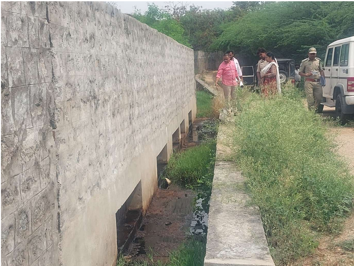
Pic 5 – Inlet of the box drain through which wastewater from the adjacent municipal dump yard enters the drainage system
