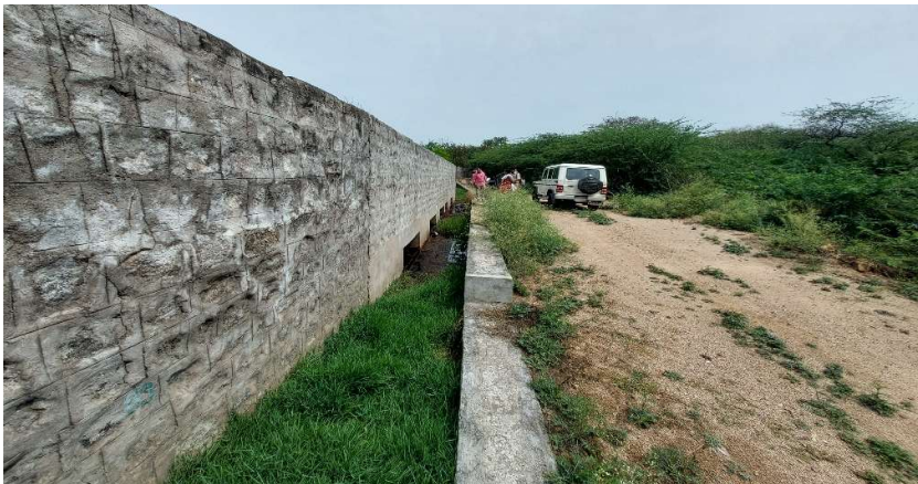
Pic 8 & 9 – Drainage canal constructed along the compound wall inside to channelise rainwater runoff into the box drain
