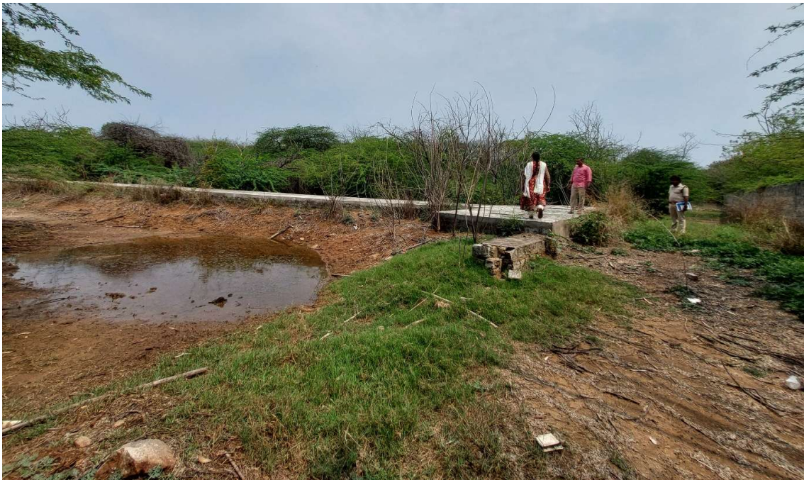
Pic 3 – Terminal end of the box drain from where an underground pipeline channels the wastewater to the CRIDA campus
