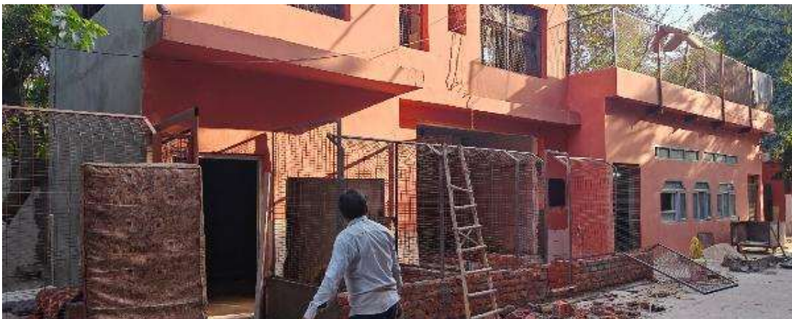
Pic 7 – In-Patient ward under construction for small animals
