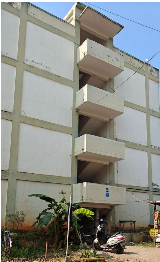
Pic 17, 18 & 19 – Views of residential apartments in Vambay colony and the JNNURM township in Ajitsingh Nagar
