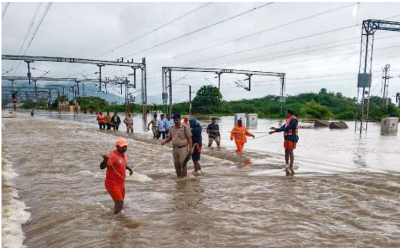
Pic 6 – Railway tracks damaged by flooding; stranded people rescued by SDMA team and Fire Department personnel
