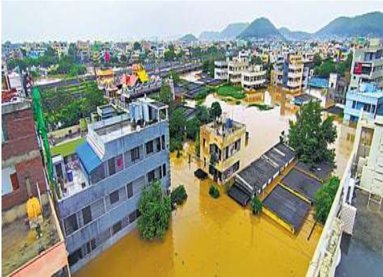
Pic 5 – Residential colonies in Ajitsingh Nagar submerged in the floodwater
